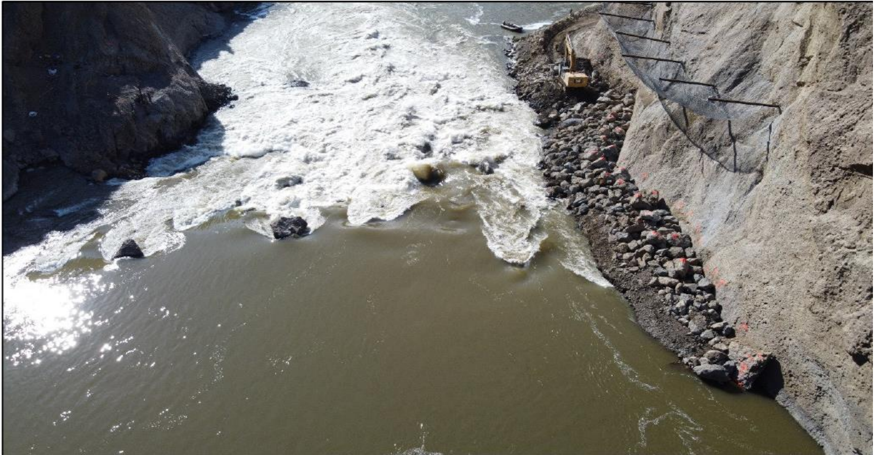
SNC – Aerial Image Looking Downstream @ West Bench Rip Rap & Select Boulders
