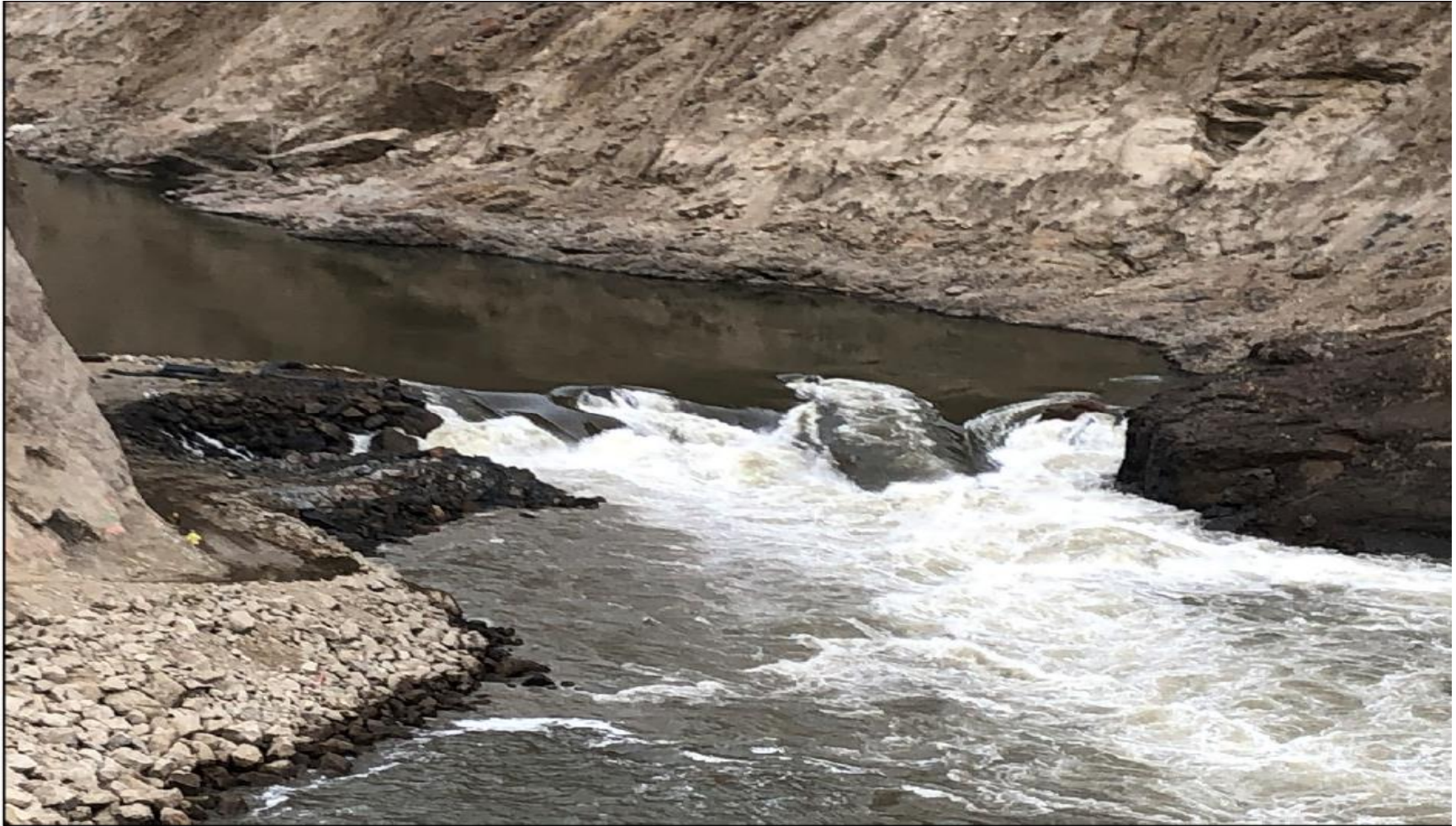
SNC – Flow @ Slide Site Immediately After M9 In-River Boulder Blast (Flow 564m 3 /sec @ 5pm)
