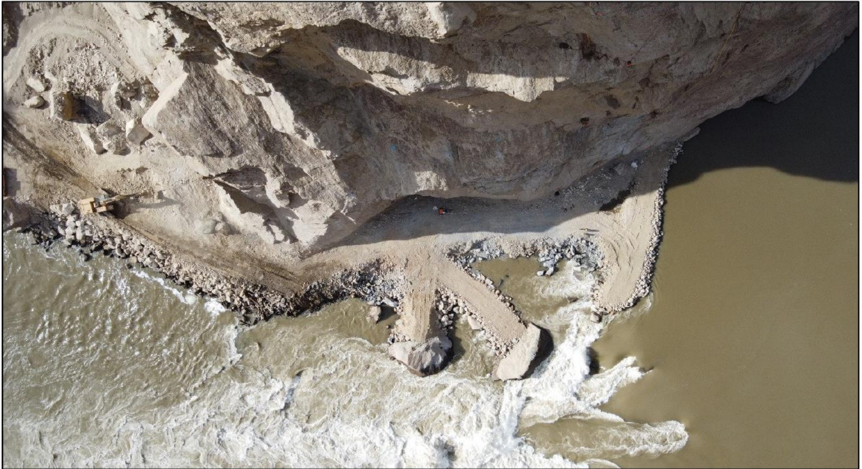
Kiewit – Aerial Image of the Slide Area & Fingers Built to Access the Large In-River Boulders (south finger removed)
