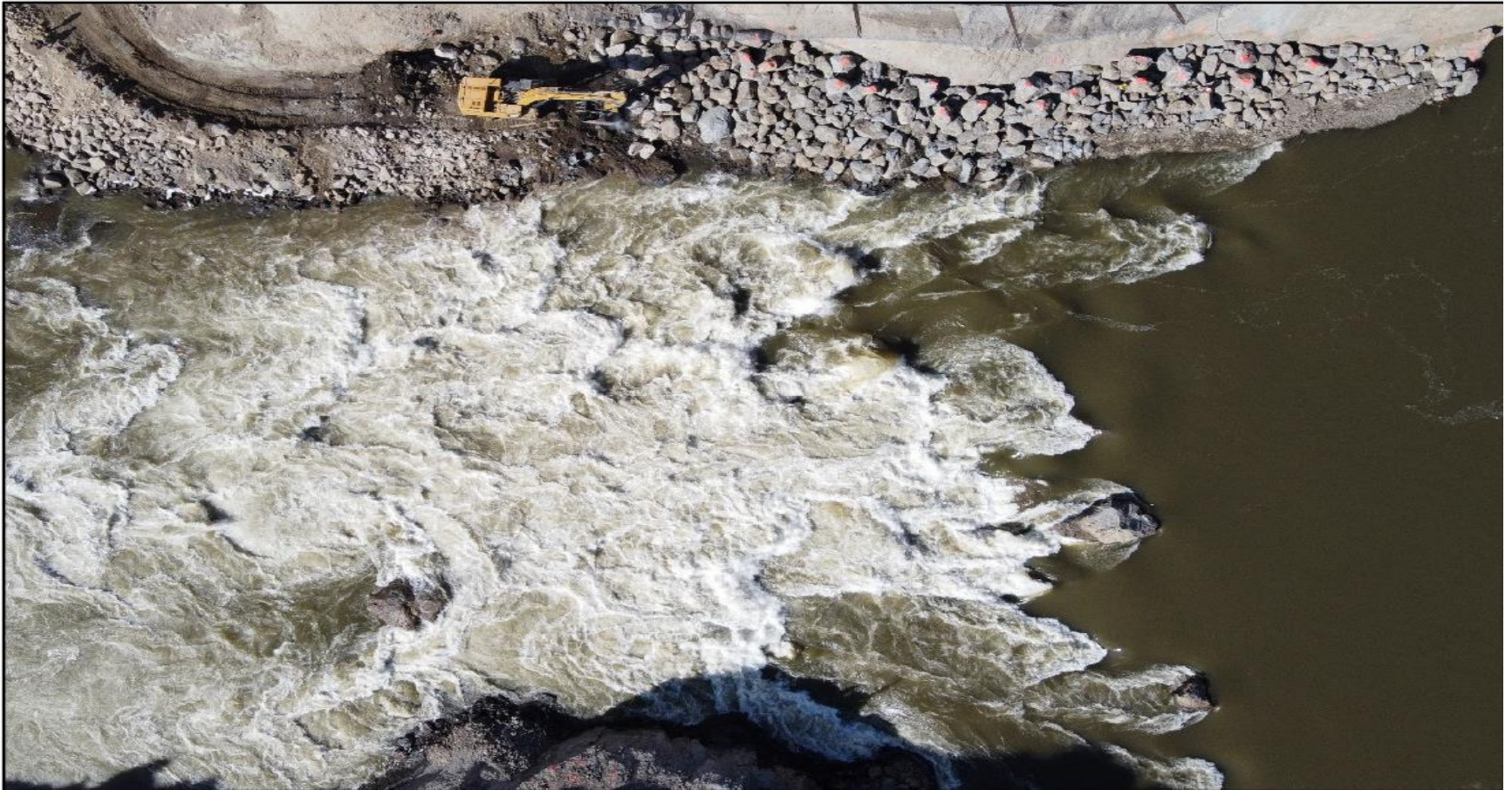
Big Bar Landslide – West Bench Natural Fishway Construction & In-River Excavation (2020-03-25)
