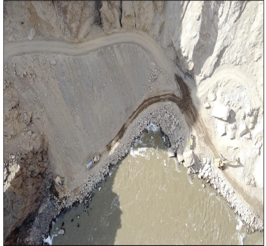
Kiewit – Aerial Image of Overland West Access Embankment Armoring Operation Sta 1+240 to Sta 1+440 approx.
