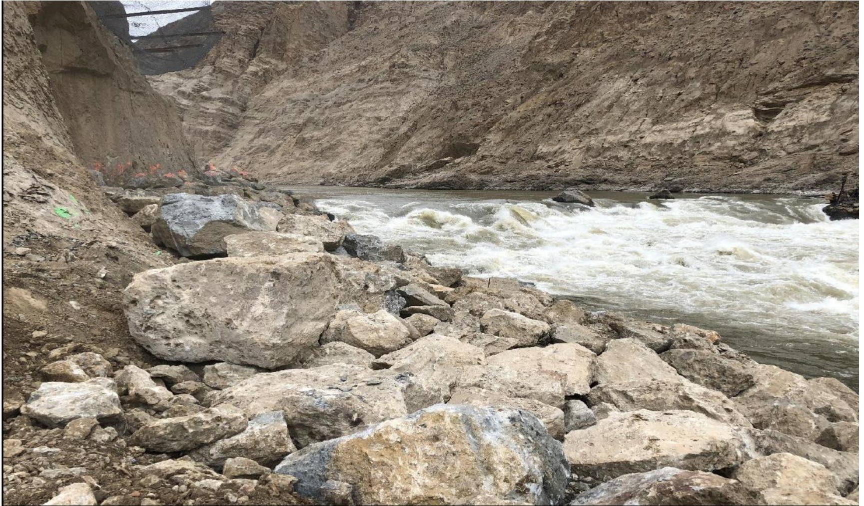
Kiewit – West Bench Natural Fishway Rip Rap Looking Upstream from Sta 1+465 (Completed Today)
