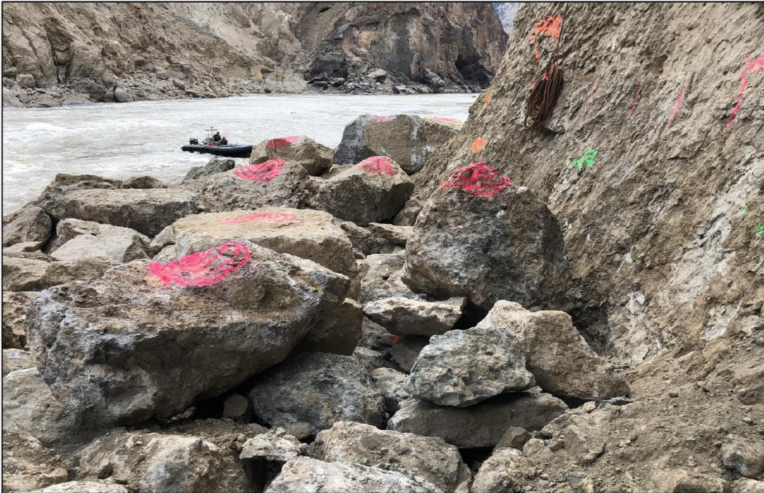
SNC – Sta 1+493 Looking Downstream @ Select Boulders on West Bench Natural Fishway (Select Boulders Marked with Paint)
