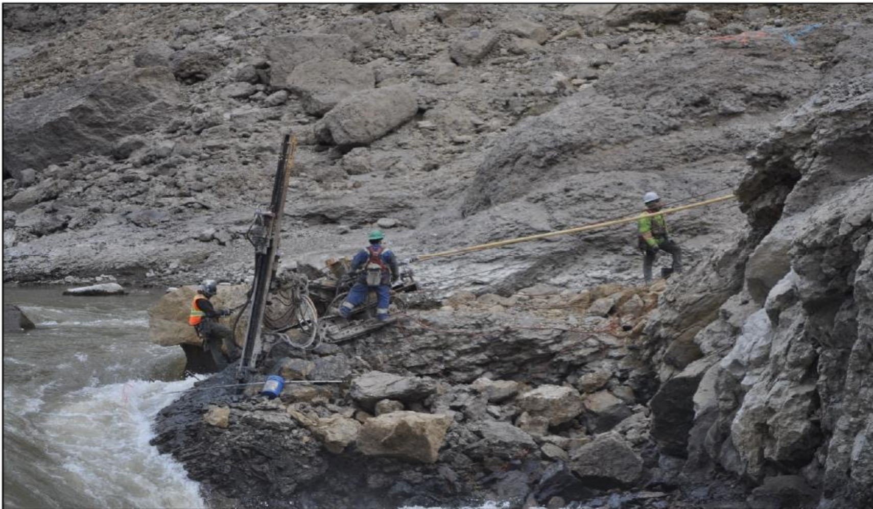
Pacific Blasting – Air Track Drilling on East Toe Upstream Rock Outcrop Previously Blasted
