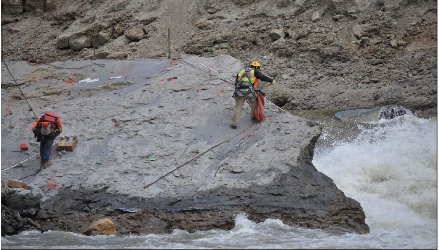
McCaws Drilling & Blasting – Loading M9 In-River Boulder for Blast
