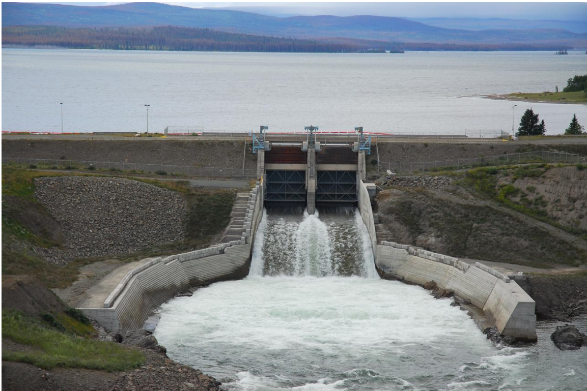
Photo: Skins Lake Spillway Photo provided by Alcan.
