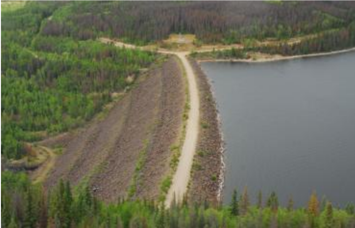
Photo: Kenney Dam
