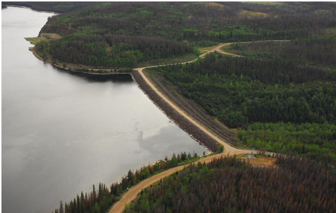
Photo: Kenney Dam Photo provided by Alcan.
