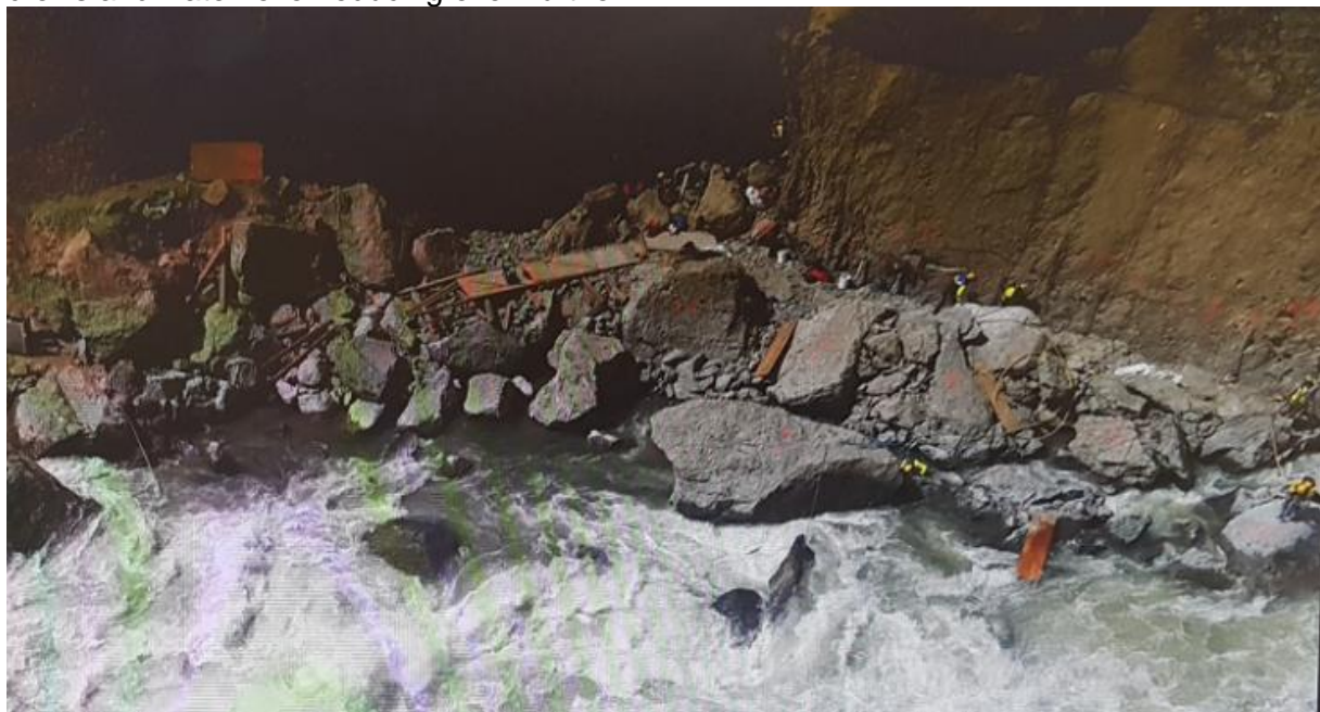
Photo 2. Fraser River at Big Bar land slide on 27 August 2019 – Discharge at Big Bar was about 2000 m 3 /s. Crews were able to safely access an large area. The work was successful. As of 3 September salmon passage was restored due a combination of instream works done by these crews and water level reducing even further.
