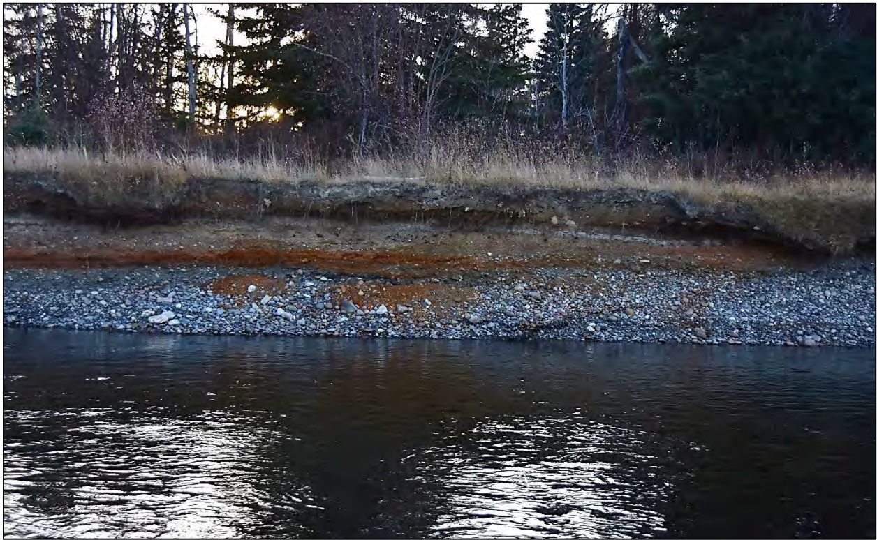
Photo 4.1 Gravel input to the Nechako River from right bank erosion at XS 223.
